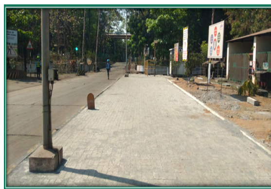
Dust Emission control by laying in house manufactured paver blocks
